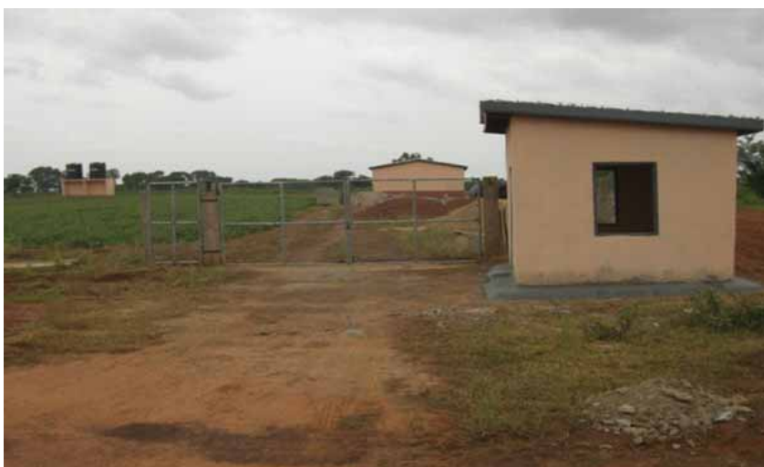
The completed CFT site at SARI, Tamale, Ghana.
