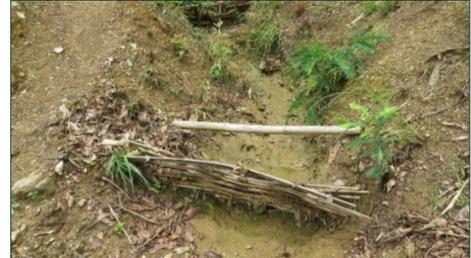
**Figure 3-7. Water from siltation pond flowing to the main harvesting pond.**
