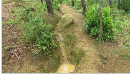
**Figure 3-6. Water channel with bamboo check dam made to control soil erosion.**
